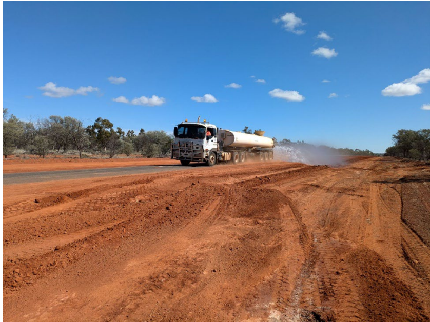
Shoulder works on 93A Diamantina Development Road (Charleville-Quilpie)
