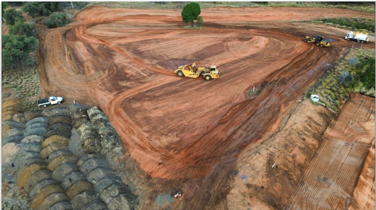
Works on the Sewerage Treatment Plant Augathella
