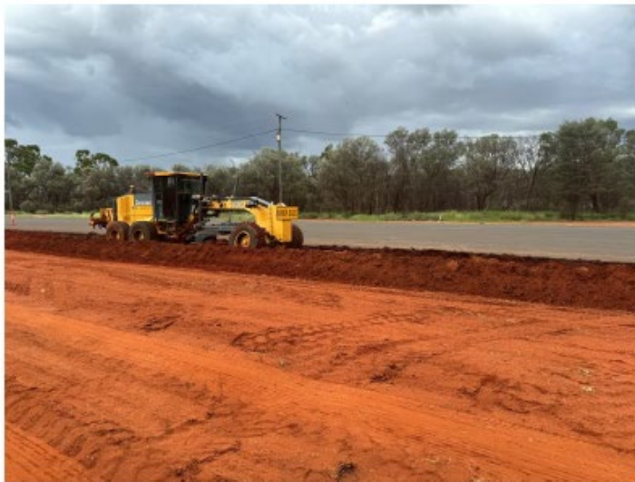
Working at the Charleville Truck Wash site and Slashing of the Landsborough Highway.
