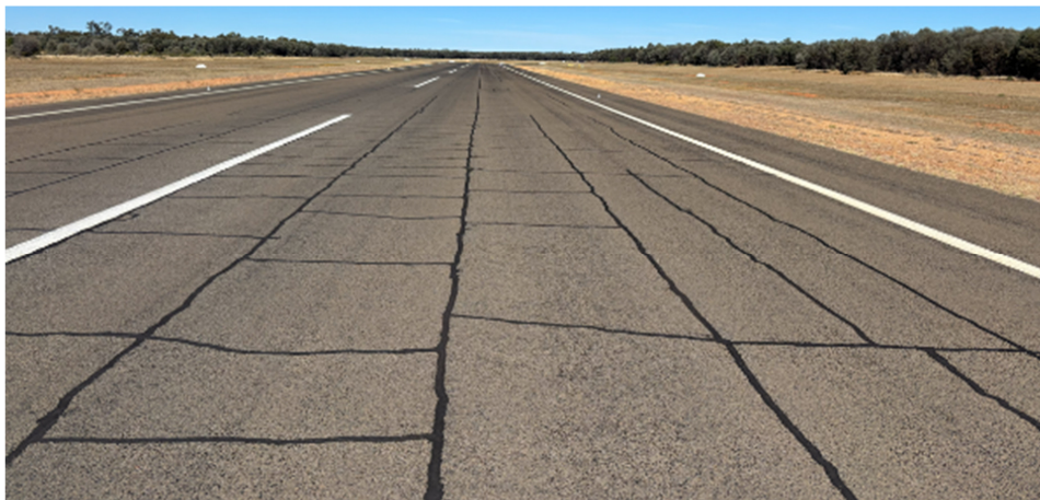
Block cracking in RWY 18/36
